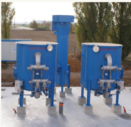
ACTINA PACK being installed on-site
